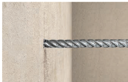
Bohren in Betonwand
