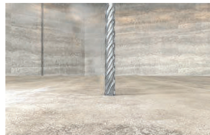
Bohren in Bodenplatte
