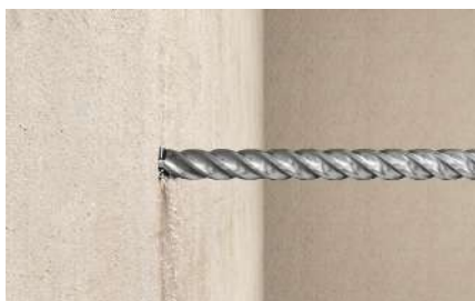
Bohren in Betonwand
