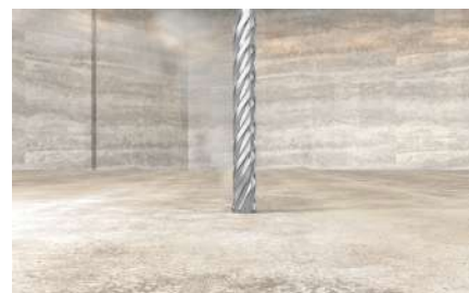
Bohren in Bodenplatte
