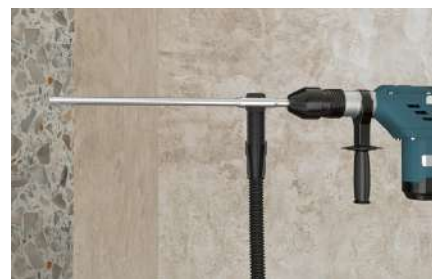
Bohren in Beton
