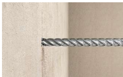
Bohren in Betonwand
