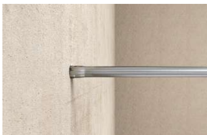
Hohlbohren in Betonwand
